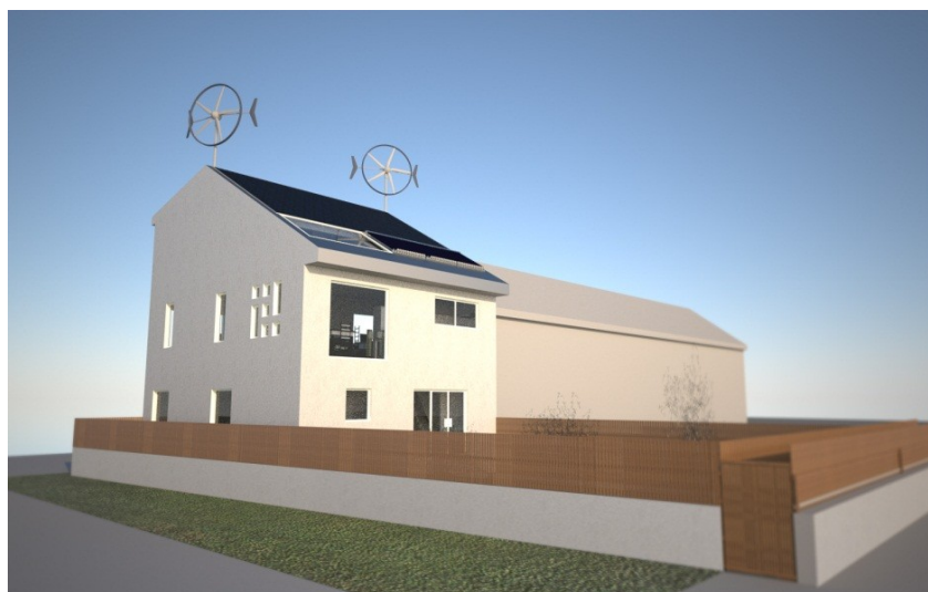
Figure 1. ZEMCH 109 equipped with a south-facing photovoltaic/thermal (PV/T) roof.
