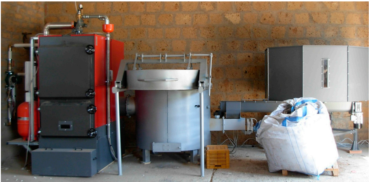
Figure 1. The biomass plant from the right side: the tank, the gasifier, and the boiler.
