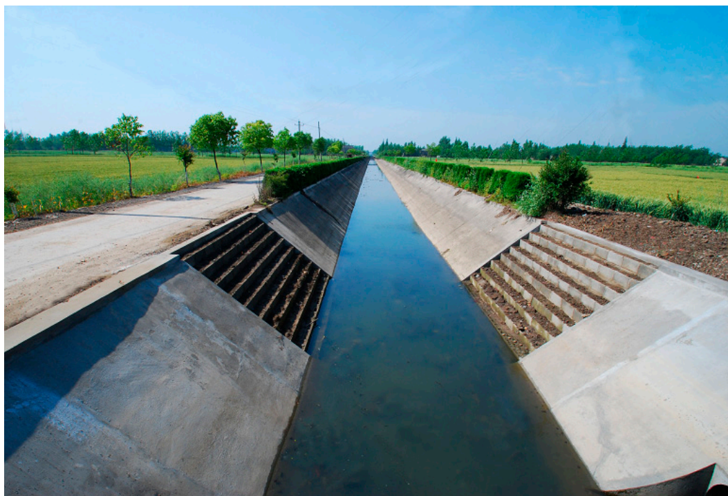
Figure 1. Escape paths for wild animals along irrigation canal slope sides in Gaoyou Irrigation District (GID).
