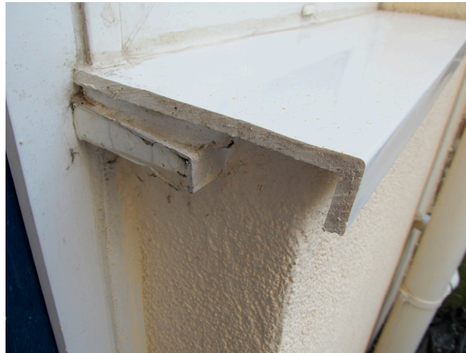
Figure 9. Fitting a new sill over existing sill.
