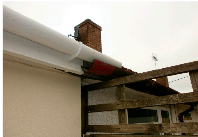
Figure 12. Undertaking works on adjacent properties.
