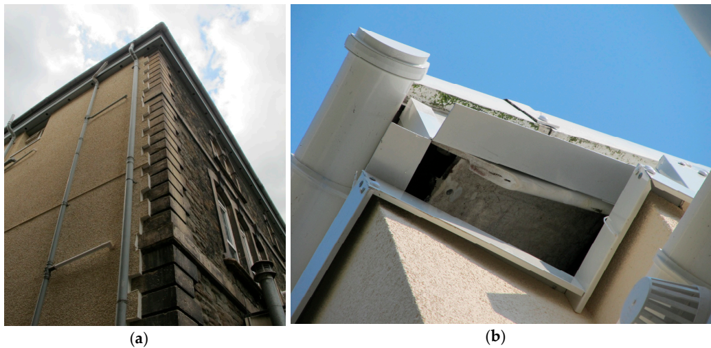
Figure 7. Difficulties when dealing with solid walled properties with intricate detailing. (a) Stone front façade to remain, with EWI having to be cut around detailing on side aspect; (b) Poor detailing around roof/wall junction.
