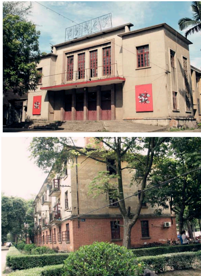
Figure 4. Guitang's community Soviet-style architecture: Movie Theatre (top) and Residential Building (bottom). Photo Copyright: Zhi Li, 2014.
