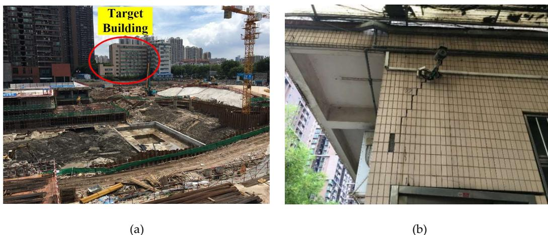
Figure 7. Photos of the analyzed building. A large foundation ditch is present on the south of the building (a). Cracks are visible on the building (b), confirming our analysis from InSAR data.
