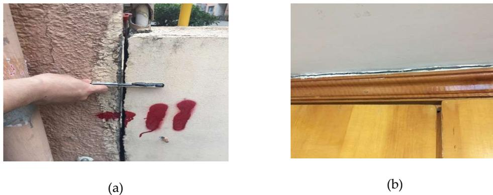
Figure 12. The big cracks (a) outside and (b) inside the building.
