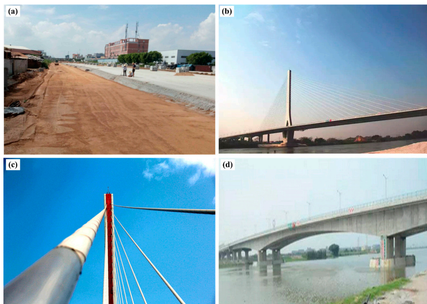
Figure 3. Site pictures: (a) Soft clay subgrade along the test highway; (b) Ronggui bridge with central iron embankment tower; (c) Enlarge picture of the iron tower in (b); (d) Anlite Bridge.
