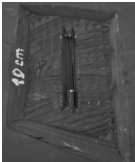
Figure 7. Example of the damage induced to the conveyor belt.
