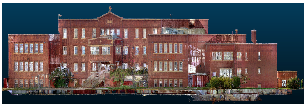
Figure 10. Old Sun Residential School: captured point cloud.
