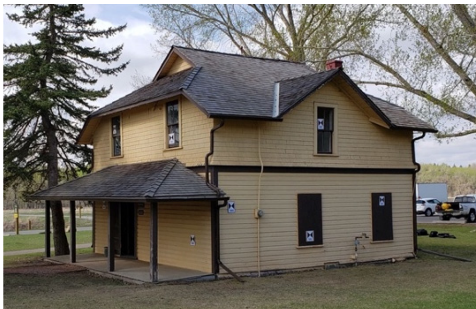
Figure 9. Jobber's House, Fish Creek Provincial Park.
