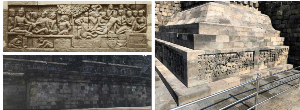
Figure 9. The example of the old photo (left top), the stone wall covering the hidden reliefs (left, bottom), and the southeast corner with the remaining four “Karmawibhanga” reliefs (right).
