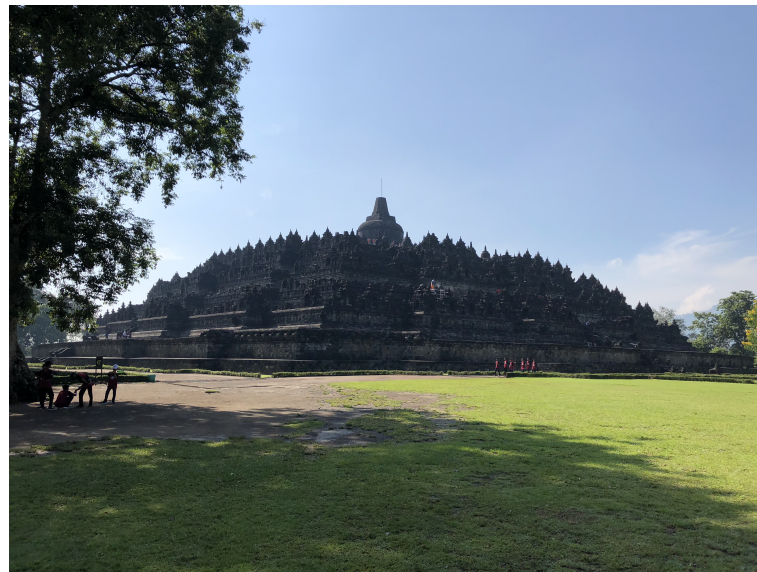
Figure 1. The Borobudur Temple in Indonesia (photograph). The entire temple consists of a series of concentric terraces of decreasing size that rise like steps to a central peak. The first and lowest part is a square base measuring 113 m on each side [20]. The upper platforms have diminishing height and the highest point of the monument is 35 m above ground level.
