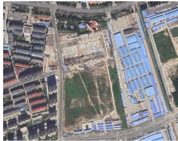
(b) Data 1: Optical image from Google Earth, acquired in 14 September 2012
