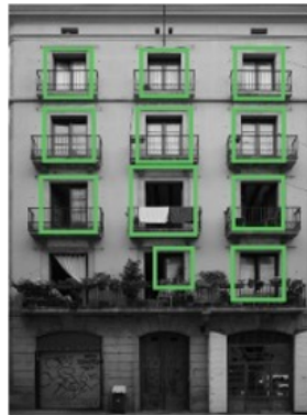
Figure 14. Example results of windows (presented as green rectangles) detected in image. Reprinted with permission from Ref. [50].
