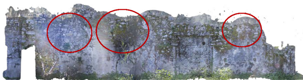
Figure 5. The orthophoto of the southern wall with the prints of the arches highlighted with red circles (authors' elaboration).
