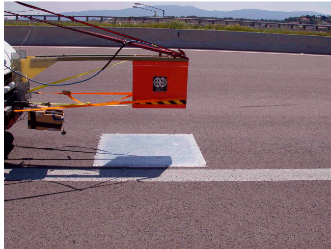
Figure 2. Determination of the incident GPR signal (copper plate placed on the pavement surface).
