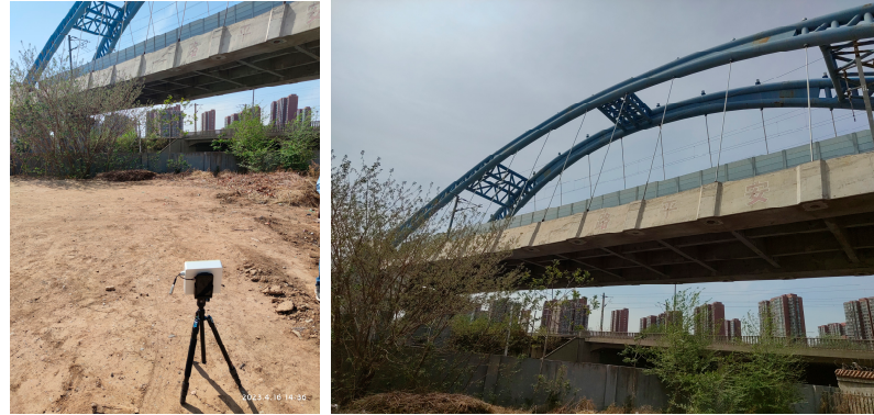
Figure 13. Photo of the bridge vibration monitoring experiment.
