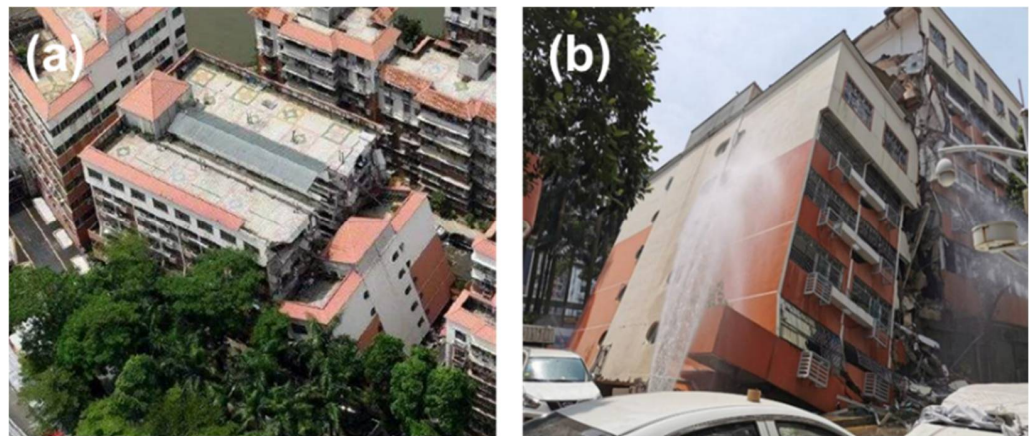
Figure 1. Site of building settlement and inclination incident: Hepingxinju. (a) Top view; (b) head-up view.
