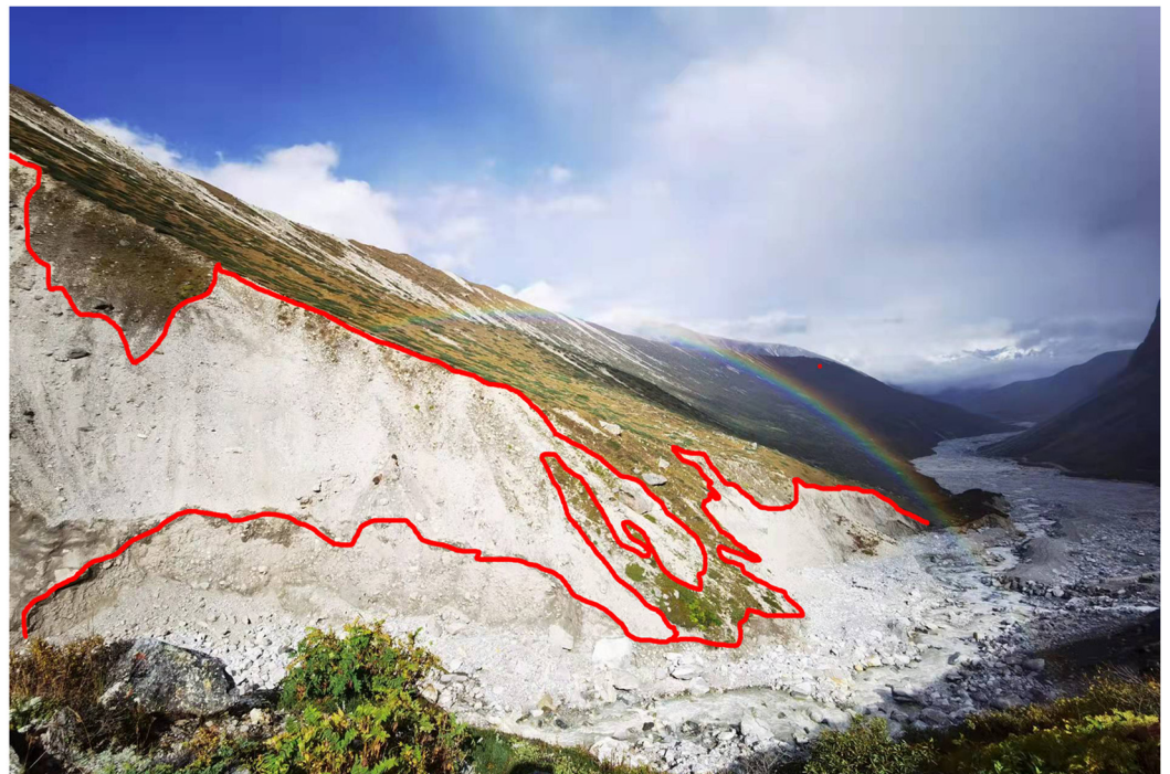
Figure 4. The slope on the opposite side of the spillway.
