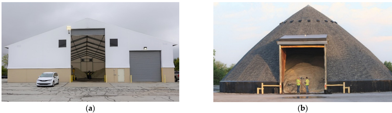
Figure 1. Samples of salt storage facilities: (a) rectangular barn and (b) dome.
