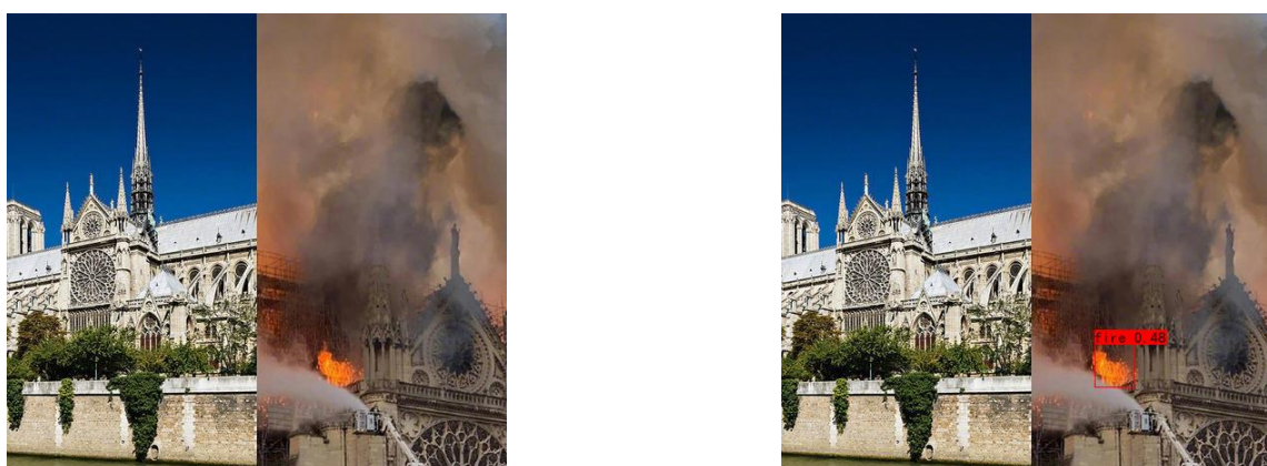
(a) Building fire
