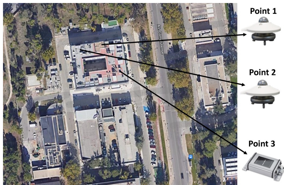
Figure 1. Image of the area under study with the building 42 in the center, including the measuring points placed on the rooftop.
