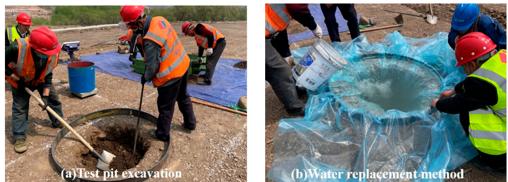
Figure 9. Density testing: (a) Test pit excavation and (b) Water replacement method.
