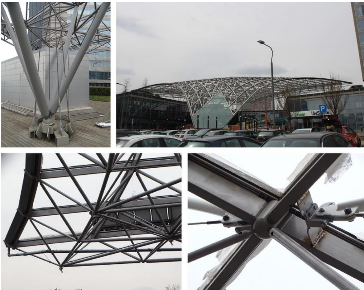
Figure 2. La Vela spatial grid structure.
