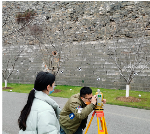
Figure 9. Surveying the cracks with the prism-free total station.
