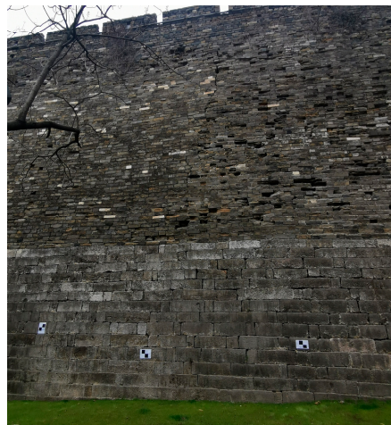
Figure 8. Part of the target points of the surveying area.
