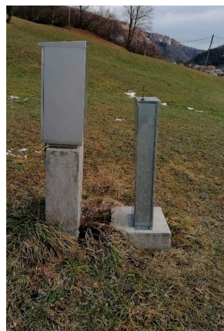
Figure 2. Measuring station used for tilt measurements.
