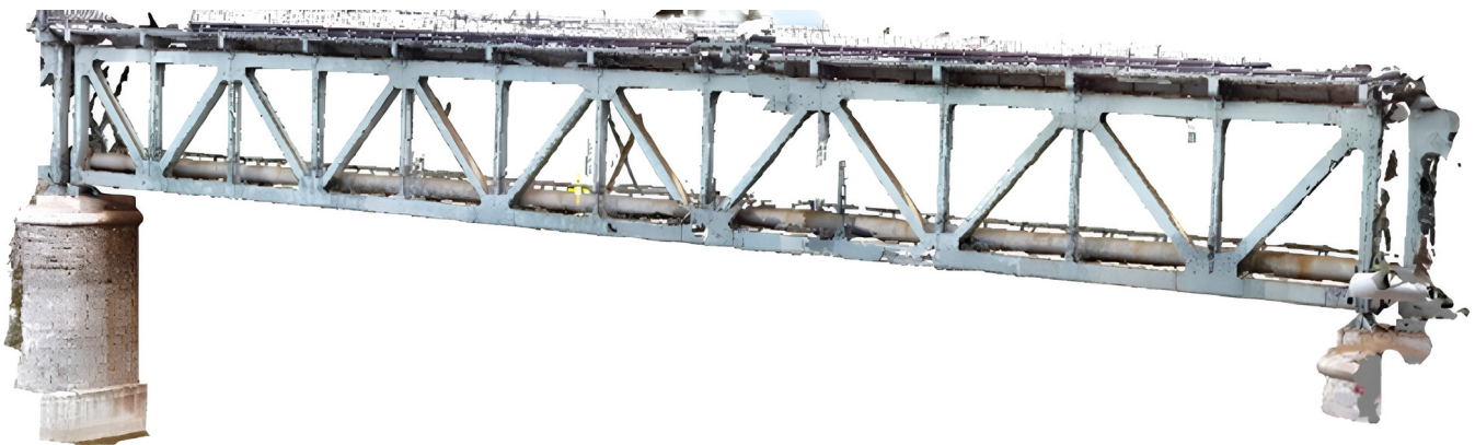
Figure 10. Photogrammetry of the inspected bridge span.
