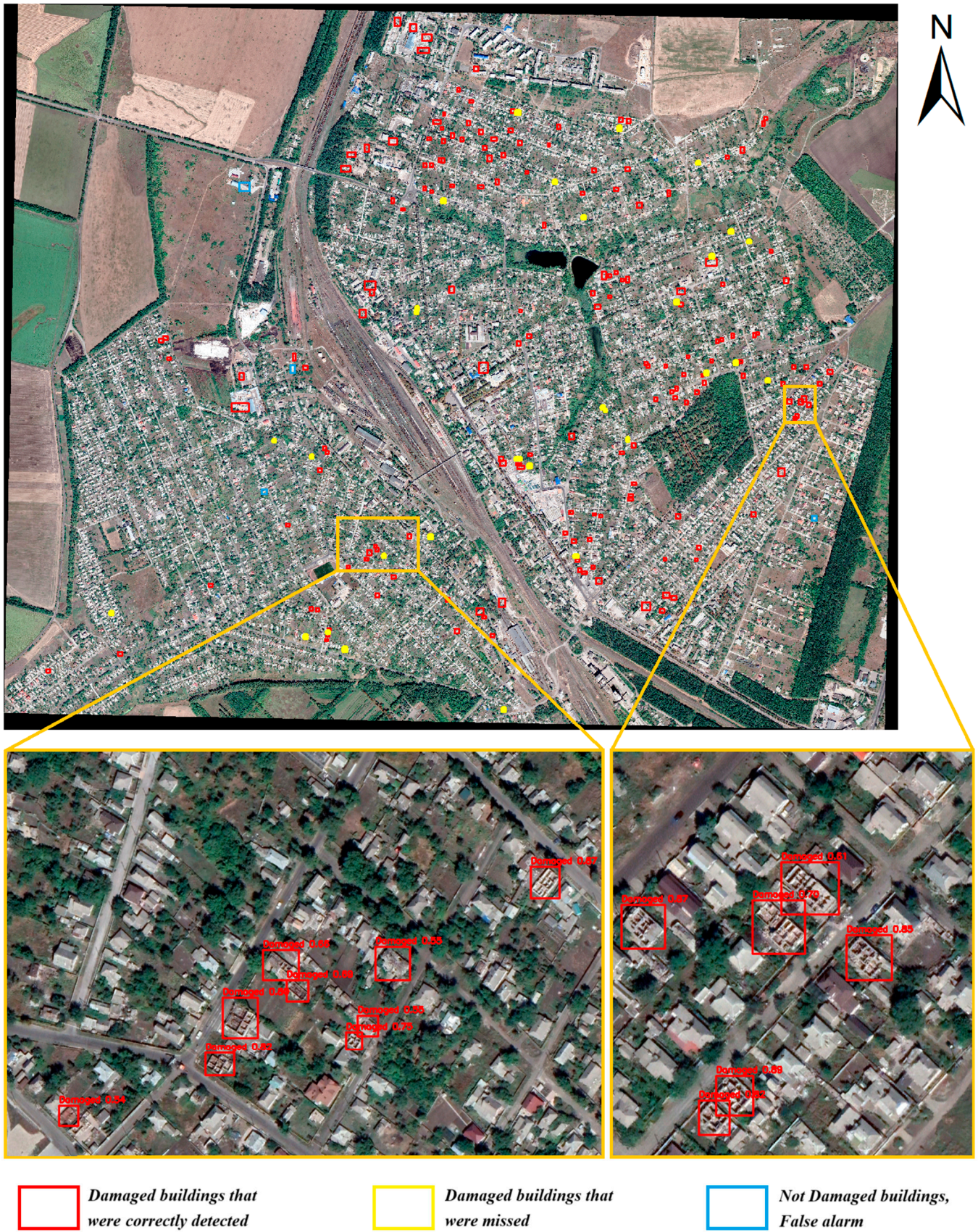
Figure 12. Detection results of destroyed buildings in Vornovakha (2 September 2022). The red boxes represent the correctly detected destroyed buildings, the yellow boxes represent the undetected destroyed buildings, and the blue boxes represent the false alarm objects.
