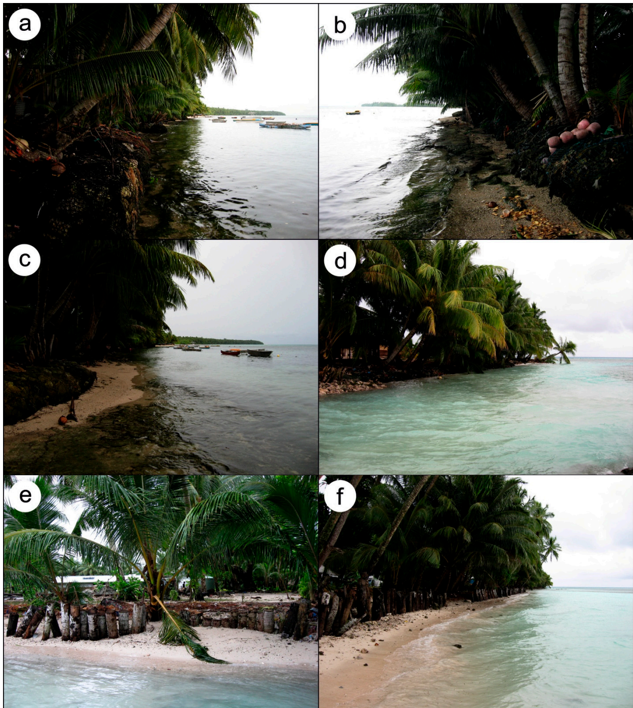
Figure 2. Pictures from seawalls on Nukutoa Island. (a–d) Traditional “rocks in net” walls (Gabion baskets). (e,f) Seawalls made of coconut logs. Pictures were taken in November and December 2008 and indicate that beach erosion prevails in front of the Gabion baskets. Photos courtesy of John R. Hunter.
