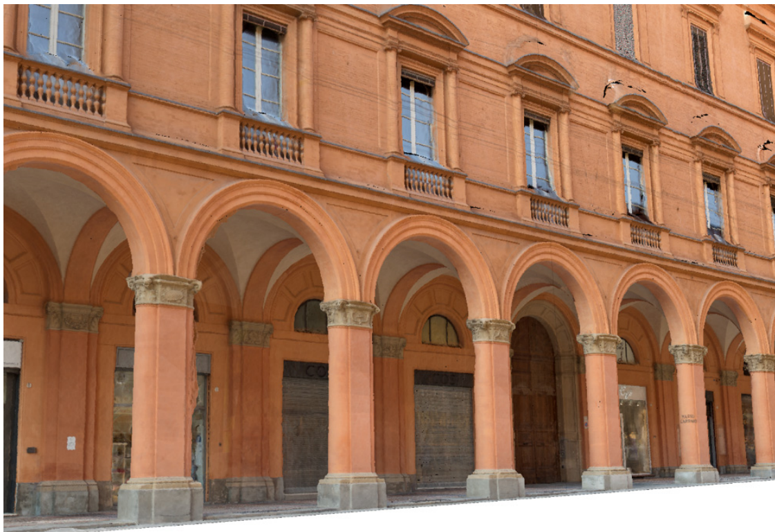
Figure 14. Example of dense 3D point cloud of a portico obtained with the presented photogrammetric methodology based on an advanced pre-processing pipeline.
