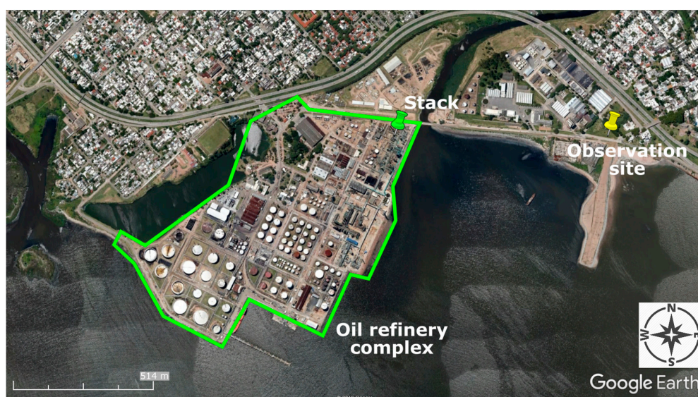
Figure 3. Measurement site (yellow marker), stack (green marker) and oil refinery facility, marked with green outline.
