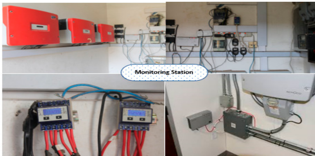
Figure 2. Monitoring station for outdoor test set-up at College of Engineering KNUST, Kumasi, Ghana.
