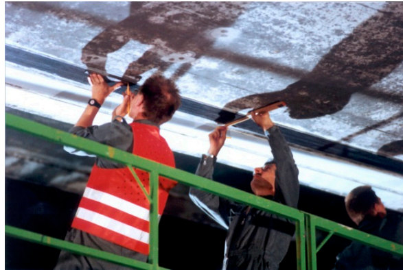
Figure 6. Strengthening work on the Ibach bridge in the year 1991.
