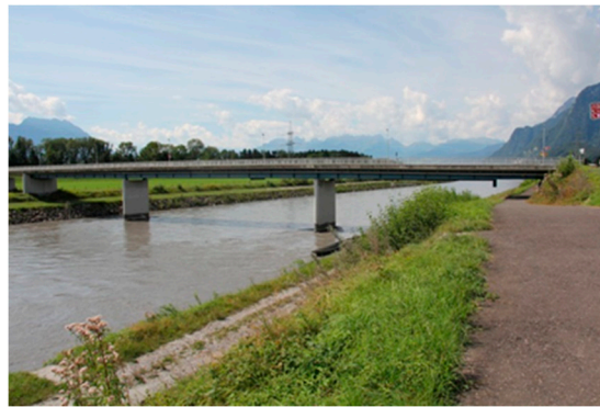
Figure 20. Bridge over the river Rhine near Oberriet in Switzerland.
