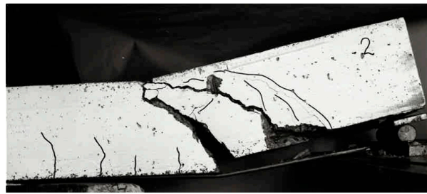
Figure 16. Failure mode in the static loading test on Beam 2B.
