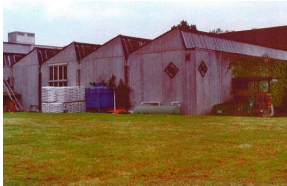
Figure 11. Industrial building in Kreuzlingen in Switzerland, which was strengthened in 1970 by means of steel plates.
