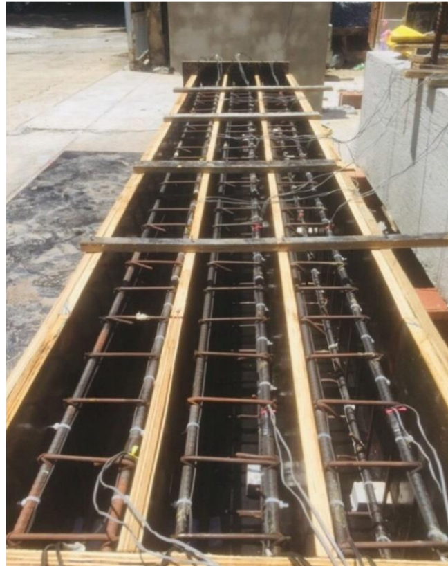
Figure 7. Application of spot glue for optical fiber bonding.
