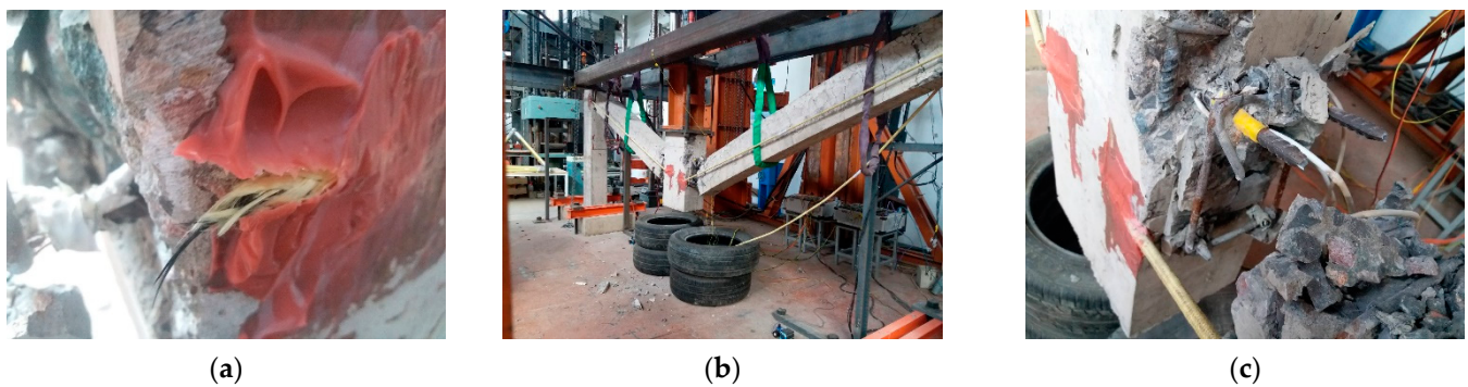
Figure 11. CFR fracture and collapse failure of the strengthened specimen: (a) CFR fracture; (b) Global perspective of collapse failure; (c) Collapse failure details at the right side of the middle column.
