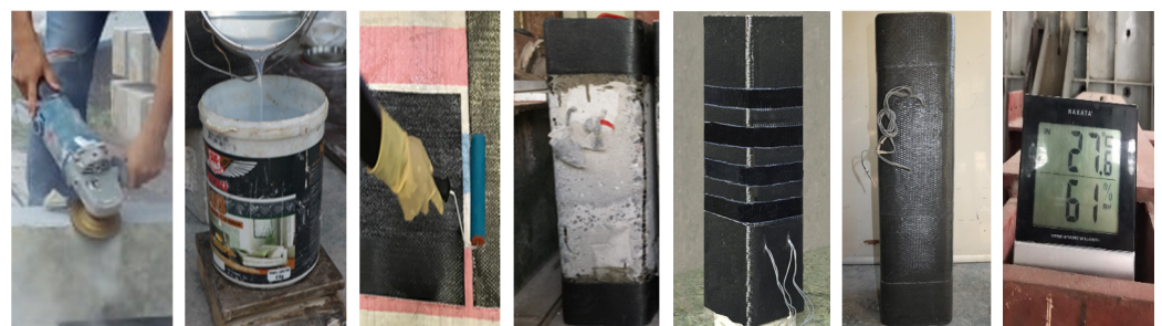
Figure 4. Procedure of strengthening with CFRP and curing.
