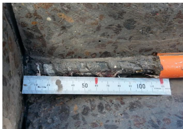
Figure 10. Steel-concrete interface on the GPC beam.
