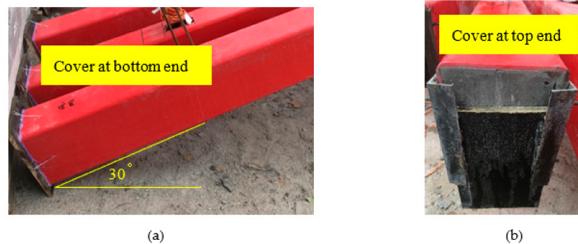
Figure 2. Casting concrete: (a) bottom end of specimen; (b) top end of specimen.
