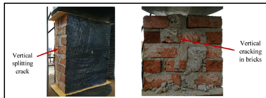
Figure 12. Failure modes of CFRP-strengthened masonry wallettes under monotonic loading (Reprinted with permission from [16]).
