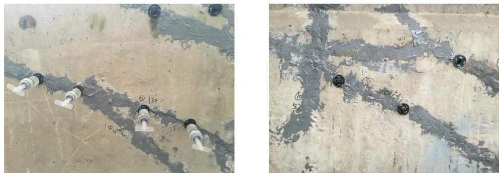
**Figure 3.** Repair of concrete cracks by filling epoxy paste.
