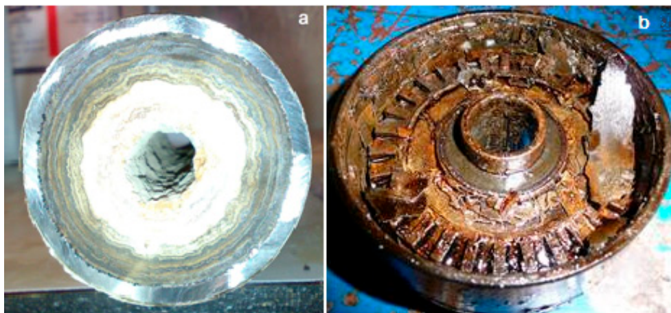
Figure 2. Calcium carbonate deposits in the pipeline (a) and the working organ of the submersible pump (b).
