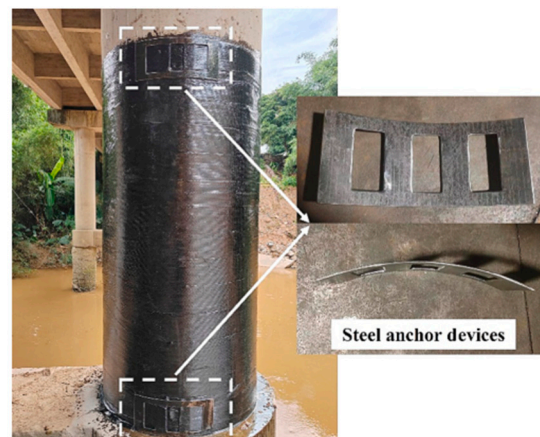
Figure 6. The bridge pier after strengthening [17].
