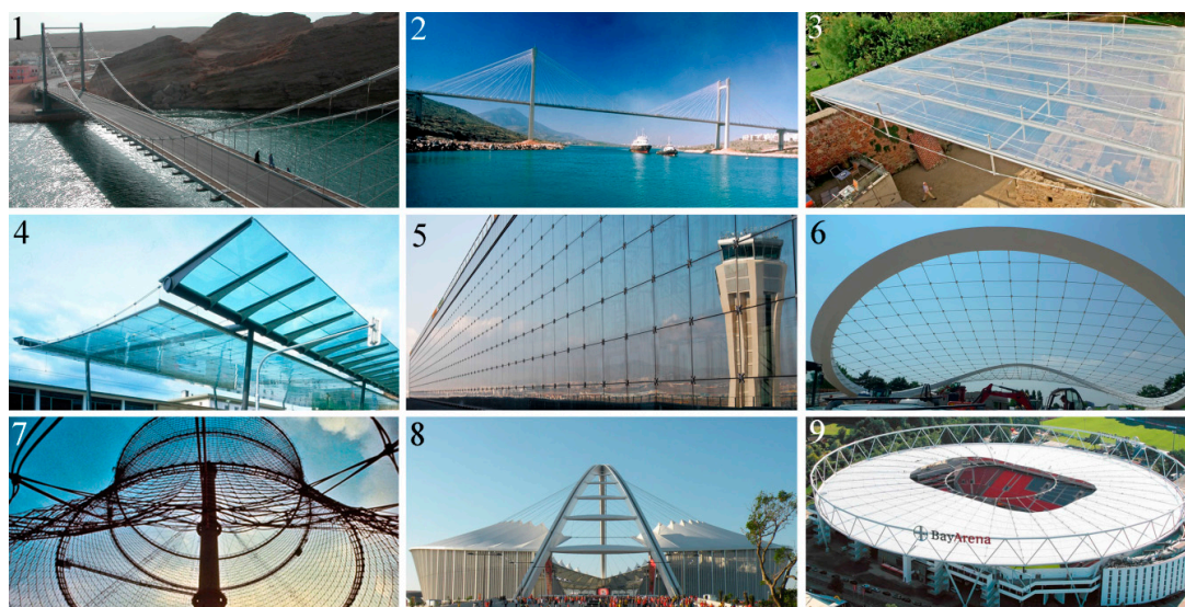
Figure 1. Typical modern cable structures with steel cables: (1) suspension bridge, Highway Bridge Khor al Batah, Oman (photo credit: STRABAG); (2) cable-stayed bridge, Evripos Bridge, Greece (photo credit: schlaich bergemann und partner); (3) cable truss roof, Annex Lutherhaus Roof, Germany (photo credit: Monika Nikolic); (4) cable suspension roof, Glass Canopy of Station Plaza Heilbronn, Germany (photo credit: schlaich bergemann und partner); (5) cable net facade, Facade Airport Málaga, Spain (photo credit: Roschmann); (6) saddle-shaped cable net, Canopy in Autostadt Wolfsburg, Germany (photo credit: schlaich bergemann und partner); (7) cable net tower, Dry Cooling Tower in Schmehausen near Hamm, Germany (photo credit: schlaich bergemann und partner); (8) arch tower cable supported roof, Moses Mabhida Stadium, South Africa (photo credit: schlaich bergemann und partner); and (9) spoked wheel cable roof, Bay Arena Leverkusen, Germany (photo credit: Bayer 04 Leverkusen Fußball GmbH).
