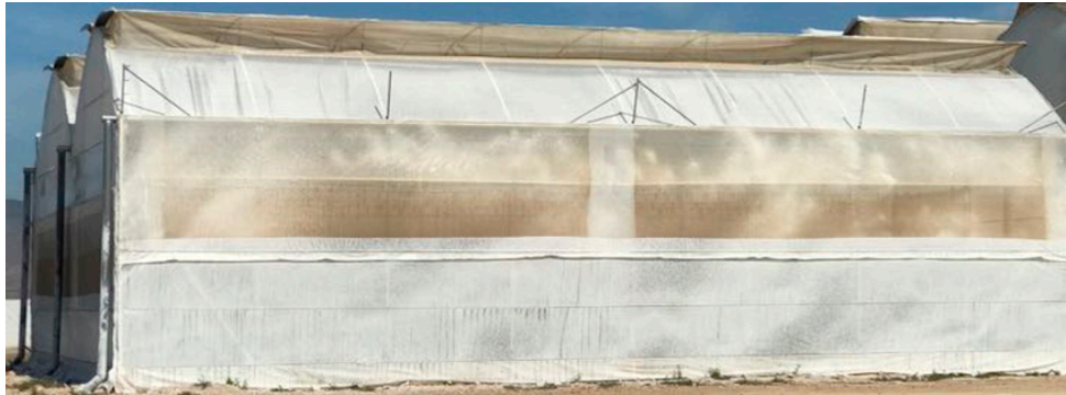
Figure 1. Greenhouse with fan-pad system.
