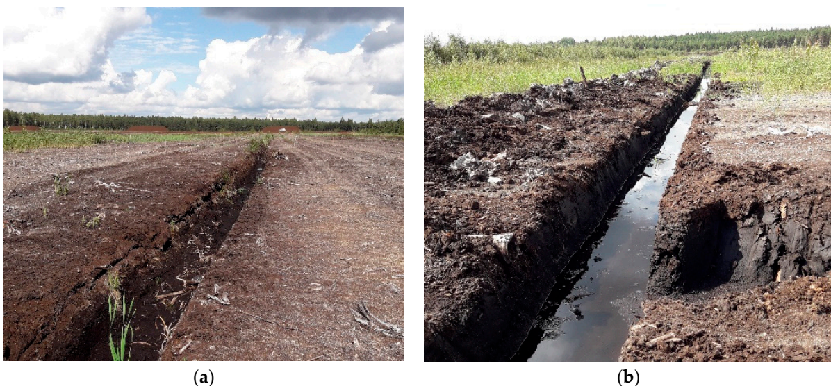
Figure 1. Drainage ditch in the study site: (a) drainage ditch before cleaning; (b) drainage ditch after cleaning.
