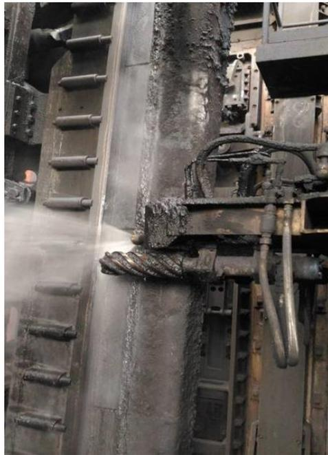
**Figure 11.** Coke oven door cleaned with a high-pressure water jet machine.
