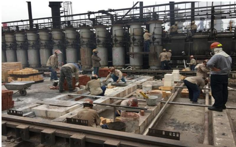
**Figure 12.** Renovation of coke oven bricks and riser pipes.
