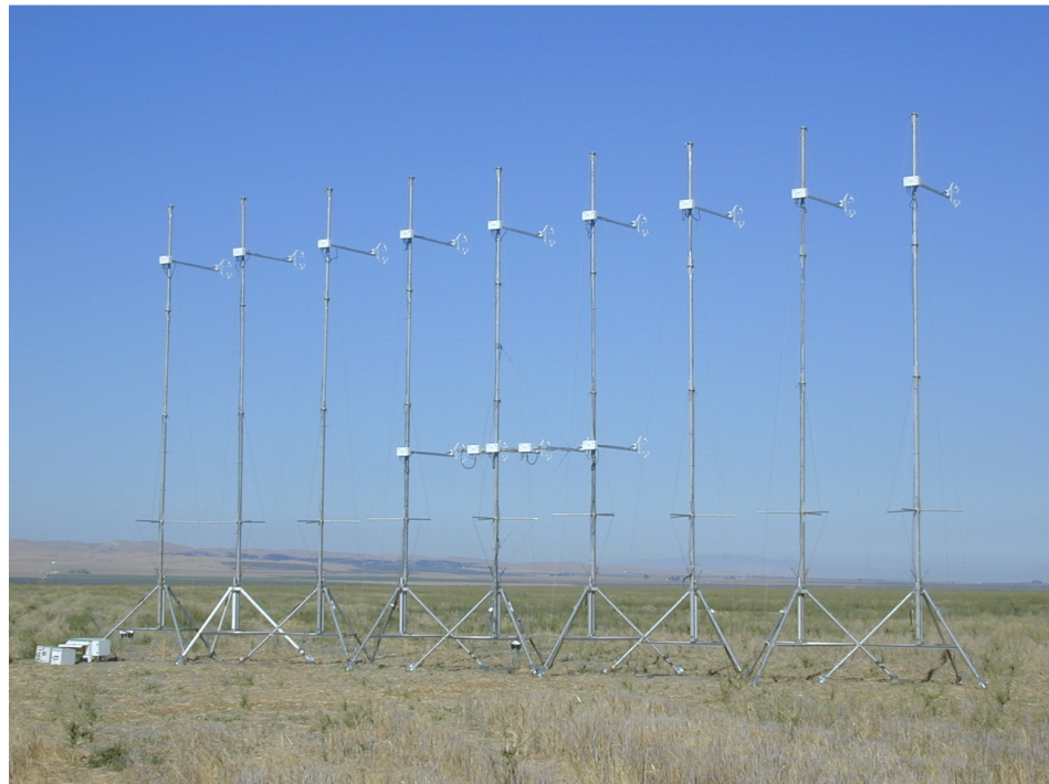
Figure 1. Twin horizontal arrays of sonic anemometers used to measure subfilter-scale variables in the atmospheric surface in the HATS field campaign. The upper array is located at z_d = 8.66 m with anemometer horizontal spacing \delta y_d = 2.17 m. The vertical location and horizontal spacing of anemometers in the lower array are (z_s, \delta y_s) = (4.33, 1.08) m. Photo courtesy of Thomas Horst (NCAR).
