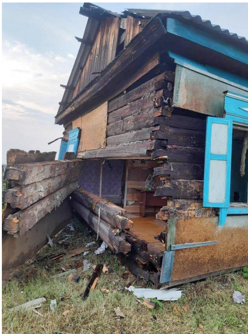
Figure 4. A wall of the house that was pushed out by an explosion of ball lightning ( https://static.mk.ru/upload/entities/2021/07/28/17/articlesImages/image/cb/6b/54/b0/fdd2dd02aeeb483cc7a2d48f8fe59e4a.jpg , accessed on 29 July 2021).
