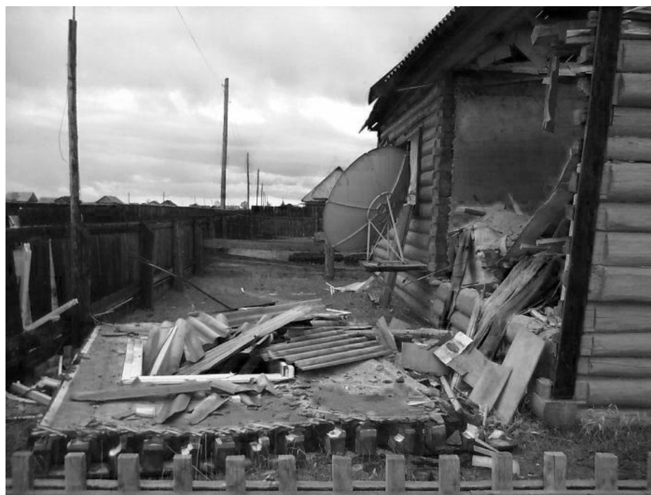
Figure 3. A wall knocked out by an explosion of ball lightning [79].
