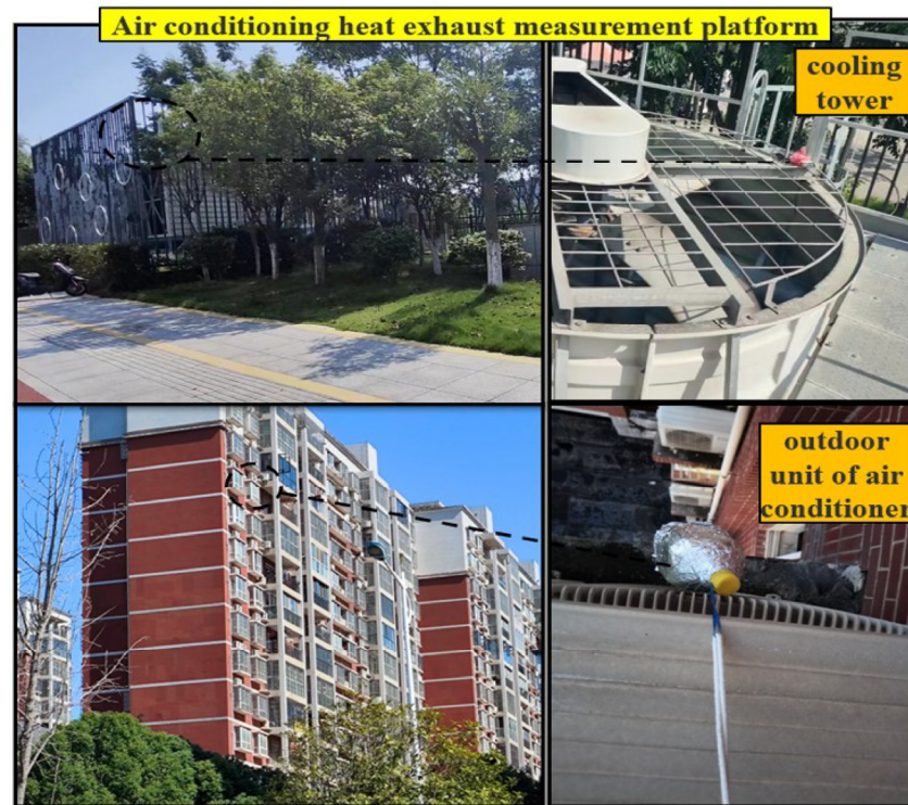
Figure 3. The measurement for air-conditioning heat rejection. The upper part of the picture shows the cooling tower measurement points, and the lower part of the picture shows the air-conditioning outdoor unit measurement points.
