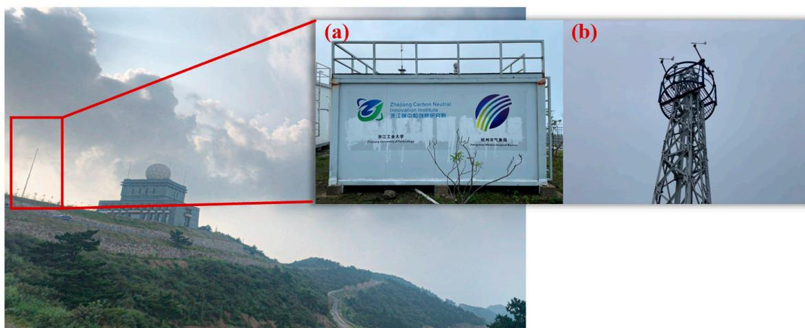
Figure 4. DMS at the hilltop flat. (a): Experimental square cabin on the summit of DMS; (b): a 10 mm O.D. sampling line outside the experimental square cabin at the top of a 10 m tower.
