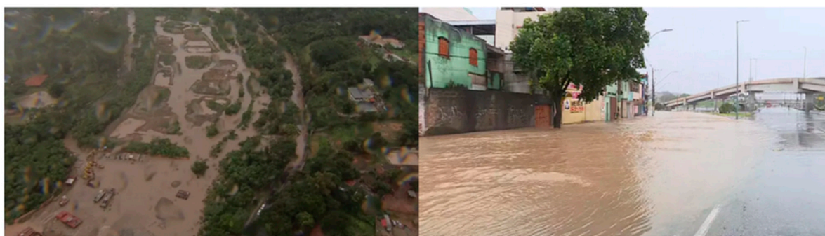
Figure 5. Photograph records of the consequences of the natural disasters’ events in Belo Horizonte on 24 January 2020. Source: G1—Photos: Reproduction/TV Globo ( https://g1.globo.com/mg/minas-gerais/noticia/2020/01/24/chuva-forte-provoca-alagamento-na-pampulha-em-belo-horizonte.ghhtml , accessed on 16 January 2022).
