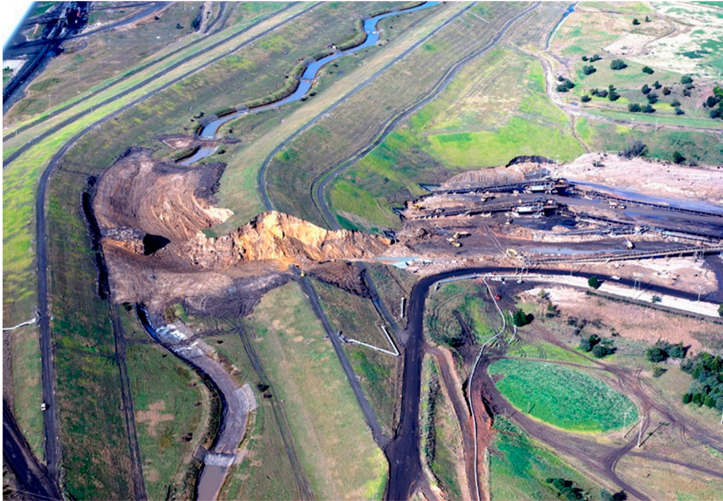
Figure 6. The 2012 Morwell River collapse. Note the meandering relocated channel and associated embankment collapse (Source: Environment Victoria).
